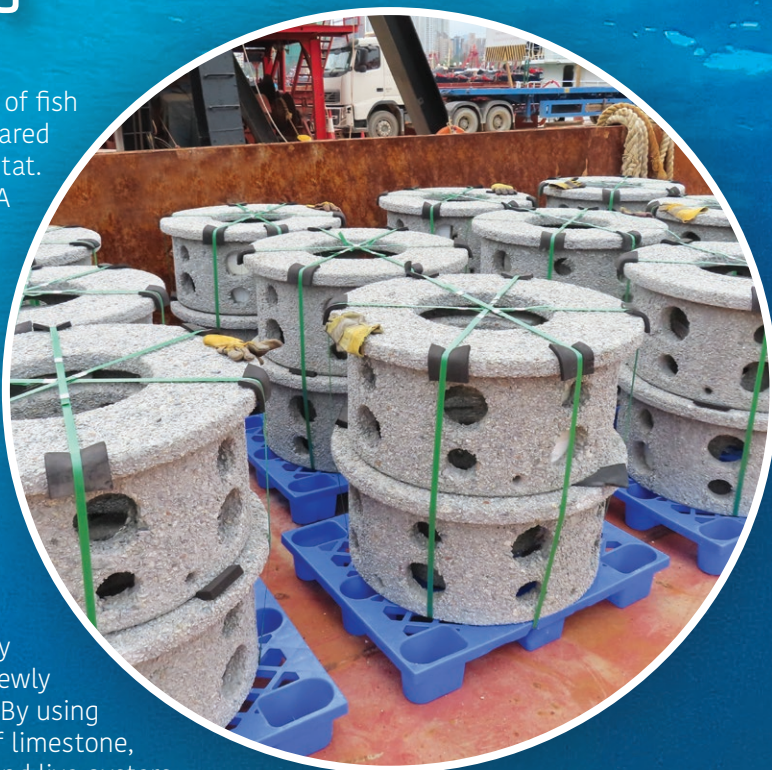
With a rough surface and holes of various sizes, the ARs encourage settlement of and provide shelters for various marine species. 人工魚礁表面粗糙並有不同大小的洞，有利各種海洋生物在此附着生長及棲息。
